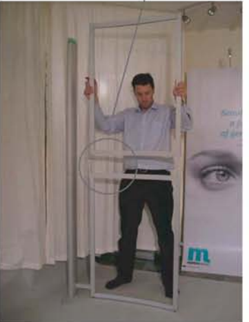
Position Upper Frame onto Lower Frame Extension Bars
